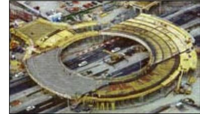
steel structure is 1.17 m and the thickness of the bridge deck is 20 cm. The beams were adjoined of three assembly sections over the dividing lane of the motorway, and then were hoisted in position at night during complete closure of the motorway, which required a total of five nights.
