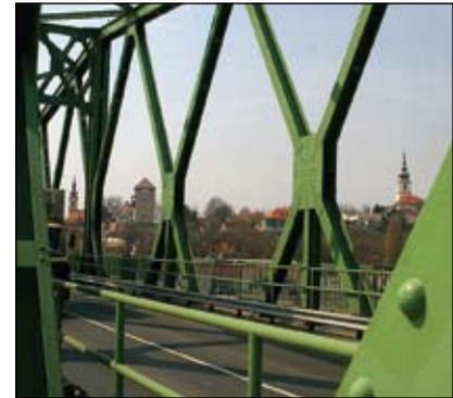
outflow side. The fact that 86 000 m<sup>2</sup> of corrosion protection coating needed to be applied, show the magnitude of the job. The plans were prepared by the Pont-TERV Co. (Iván Pozsonyi), the contractor was the Bridge Builder and Közgép Consortium (Hídépítő-Közgép Konzorcium).
