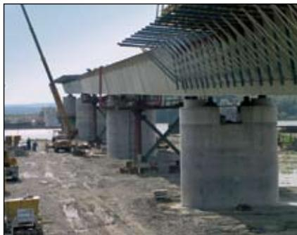
riverbed piers, 8 m wide, 16 m long and 4 m high so called shaft pieces were used. These pieces were accurately lifted in place and were secured by pouring rocks around them. The pile footings were poured via steel tubes welded in place previously, and then – once the water proofing concrete was poured – the traditional pier construction could be continued using large piece formworks in a dry area.
