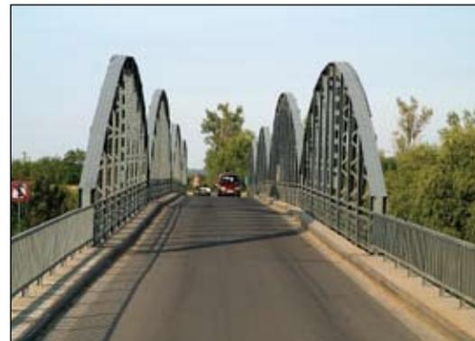
was strengthened with such a method that the upper cross beams were not necessary anymore. This way the bridge became more airy and most importantly safer for drivers.
