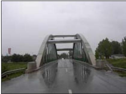
In 2003 the construction of the road section bypassing the city was begun, as a part of which an arched bridge was planned where the road intersected the river Rába so as to serve as a preliminary study of the Danube-bridge at Dunaújváros.
