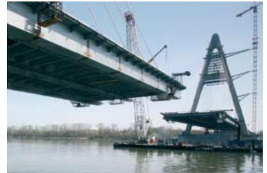
The front cover shows the Pentele Danube-bridge built in Dunaújváros in 2007; its riverbed span is the largest (304 m) in the world amongst the basket-handle arch bridges.
