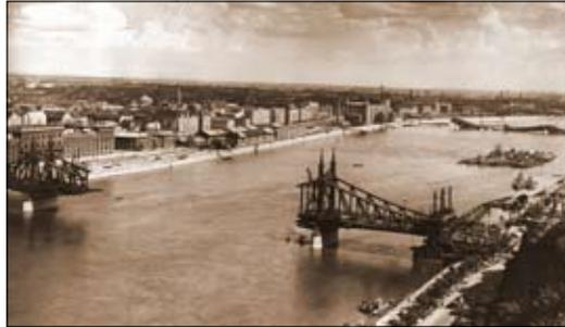
row for two tram tracks and one traffic lane in each direction. The structure of the main girders made it necessary to add 600 tons of counterweight nearby the abutments of the bridge on each side.
