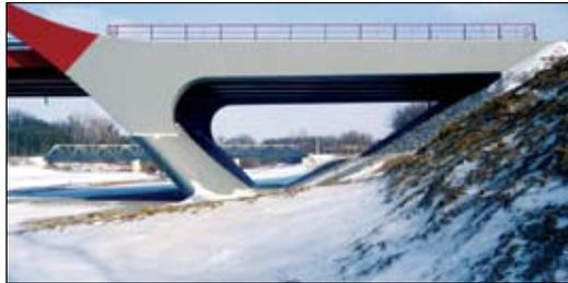
Because of the complicated technology, the ascending walls of the aesthetically pleasing and nationwide unique geometric riverbed piers were poured with self-compacting concrete.
