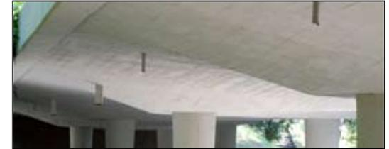
when approached from any direction, with the outward ascending distorted surfaces on the bottom of the deck and with the wavy surfaces dividing these. The detailed static calculations of the novel structure were prepared by Egon Éliás.
