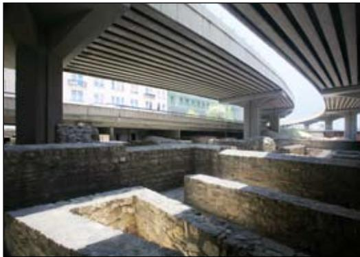
Two detached bridge structures were built for the traffic route of Szentendrei Rd. – Árpád Bridge. Because of the circumstances of the location the layout of both bridges is curved, with a smallest radius of 150 m, to which a perfect connection could have been made with the application of post-stressed box girder structures. However, due to construction difficulties a decision was made to apply custom altered EHGT-beams.
