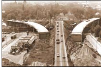
crete box shaped structures, with cross girders above the piers and at midspans. A Gerber-structured, restrictedly prestressed structure was built over the railway tracks, where it had to be ensured that the bottom surface would be crack free. The spans of the structure are between 26 and 35 m, its total length is 302 m.
