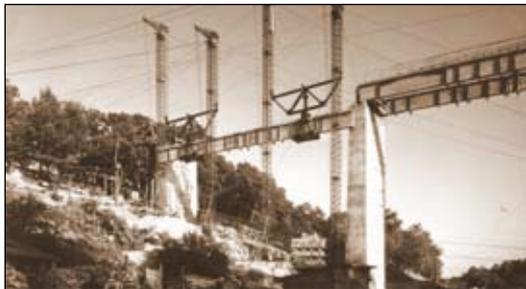
which would have simultaneously lifted the two main beams fitting into one opening. During the first lifting the beams stiffened at their top with horizontal bracing device – due to the accumulation of several unfavourable conditions – broke and fell down, pulling along the lifting devices. The accident set back the technology.
