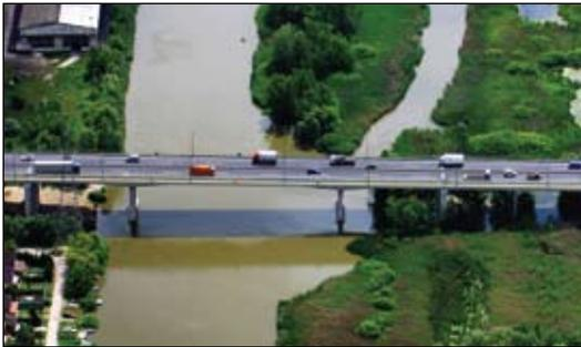
The plans were prepared by the Roads and Railways Design Co. (Uvaterv Co.) (József Varga), the general contractor was the Bridge Building Co. (Hídépítő Vállalat), which submitted the most favorable proposal for the international tender. The bridge was built between 1987 and 1990. The road is 17.5 m wide, its north side has a 3.35 m wide sidewalk while the south side has a service sidewalk.
