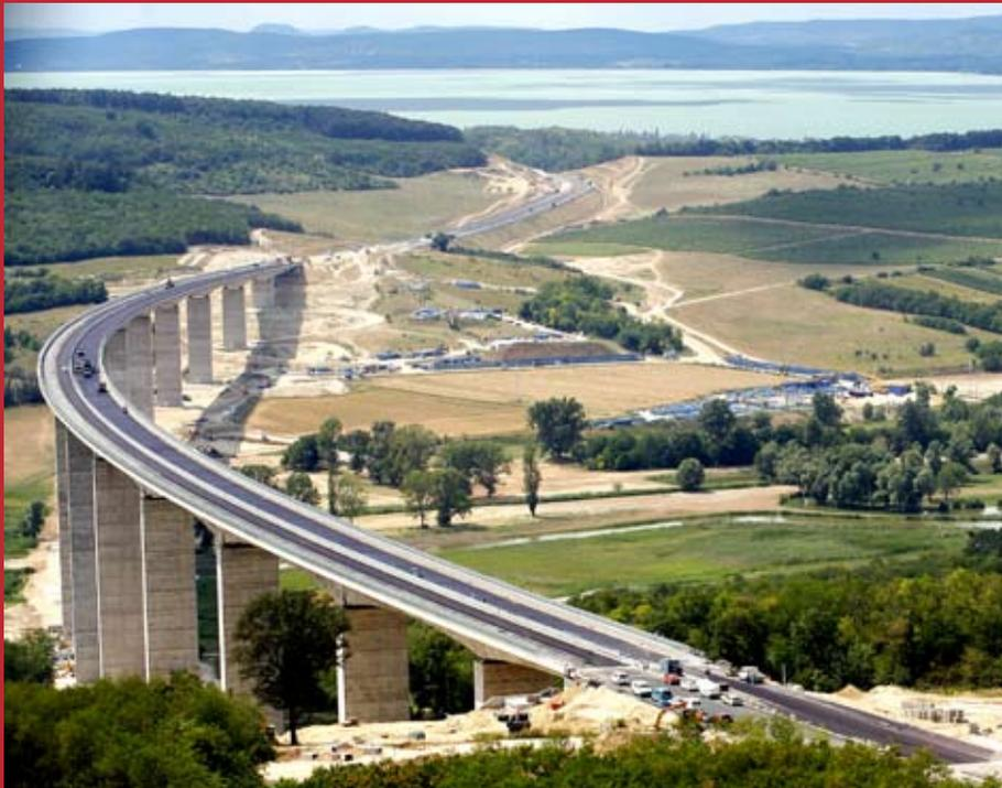
The Kőröshegy viaduct of motorway M7 built 2007 is the longest (1872 m) and highest bridge of Hungary
