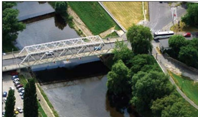
at two cross sections on March 28 of 1945, right before the last payment was made on the state loan. A temporary bridging solution was built on top of the wrecks on which traffic could run until early March of 1946 when the remnants were lifted from the river and the structure could be reconstructed using 25 additional tons of material. The welding passed the tests with excellent results.
