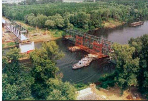
DEng and Róbert Folly became redundant. The new bridge at the outskirts of Cigánd could be built with the reuse of the 106+106 m spanned truss structure that was superfluous in Polgár. The transportation of the structure was a brilliant juggling act, since the dimensions of the delivered product were impressive. The 106 m long, 9 m wide and 10.5 m high truss structures weighed 410 tons.
