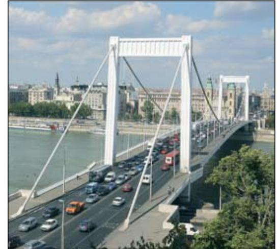
and had a larger load bearing capacity was built using about half amount of steel (6300 tons).
