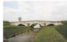
**11. Héhalom, three-span arch bridge**
