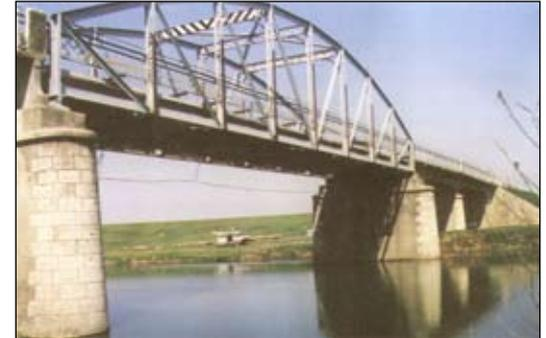
enforced. At this time a decision was made regarding the future of the bridge that the destructions caused by high vehicles need to be eliminated by removing the cross beams and the structure needs to be strengthened. An ingenious solution was applied for the renovation and the modernization as a provisory was attached to one side of the bridge therefore traffic could be kept on going during construction.
