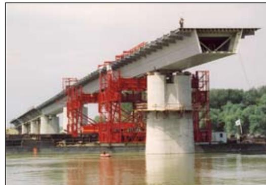
tion to the construction of the bridge at Cigánd. This technique was further developed, minimizing on site work, thus the assembly phase became more economical since considerably less prestressed bolts needed to be used to attach the sections.
