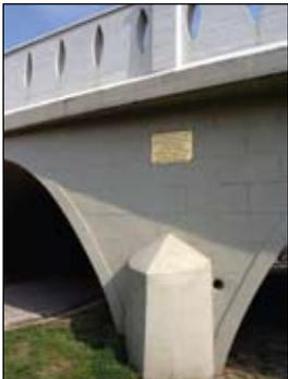
The bridge in Solt has two parabola shaped 5 m spans and a height of 3 m. The thickness of the arch is 14 cm in the middle, and 21 cm at the shoulders. The foundation of the abutments and the piers reach 120 cm deep into the good quality soil. The original grid was made of 1 cm di-
