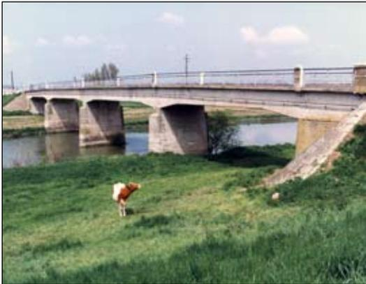
Our country was leading in the construction of the multispans continuous or hinged large span bridges, but a number of these were built outside of today's Hungarian borders or were exploded during World War II. The bridge named after Gróf (Count) István Tisza remained almost intact, only the second span from Zsadány was exploded. This was rebuilt in 1947 and thus the almost 80-year-
