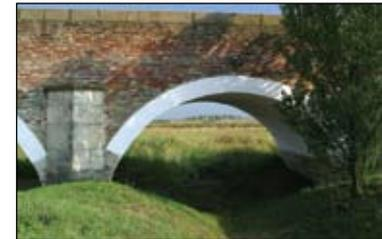
cerning the bridge. Of the original nine spans of the bridge, five – each 3 fathom and 3 feet wide – were kept, the two fallen spans on each end were dismantled, and the wing-walls were moved to the river piers on the edges of the remaining bridge section. The budget of the bridge was calculated by Fábíán Dobrovai a master mason from Abony, so most conceivably he was in charge of the renovation of the bridge.
