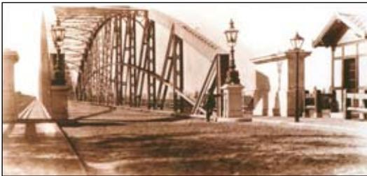
In 1891 Gábor Baross, the minister of transport approved with his signature the construction of the bridge and signed a contract with the general contractor, Gregersen and Sons. The superstructure of the steel truss bridge was manufactured and assembled by the Hungarian Royal State Wagon and Machine Factory.
