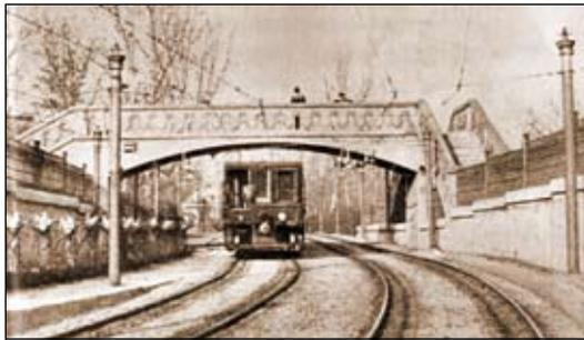
The monolith reinforced concrete arch bridge and the rest of the reinforced concrete structures of the tunnel: the parapet walls and the arches above the railway tracks were built on the basis of Róbert Wünsch's trademarked technique. The use of rigid insert structure was an important trend in the early phases of reinforced concrete construction.
