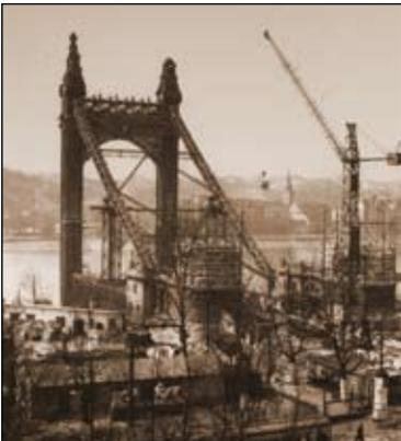
The truss-type stiffening girders of the superstructure were continuous and 44 + 290 + 44 m spanned. The 11 m wide road and the two 3.5 m wide sidewalks also were between the stiffening girders. The tram tracks used to be on the sides of the bridge road.
