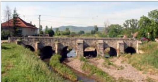
The dimensions and structure of the bridge implicate that its current shape was formed in the 18th century, by remodelling an older bridge. There is no data available regarding the construction of the bridge; however, it is believed to have been built in 1796. The total length of the bridge is 40.2 m, but its span is only 2.7 m wide. The bridge spans over a large ravine, which explains this great discrepancy in dimensions. The original arch is 8 m
